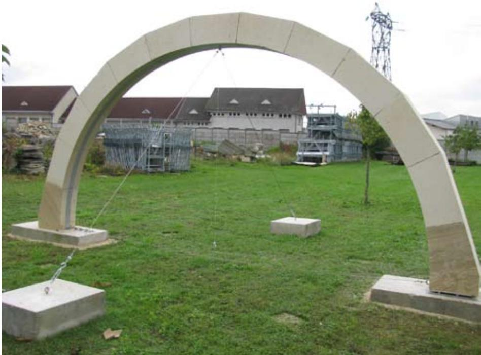
These function as the metal version of stone contact surfaces, and are sloped, with respect to the horizontal plane just like joints in an arch. The function of the steel bands is to keep the arch firm, preventing dilation of the joints and, as a consequence, guaranteeing the absolute stability of the whole structure.
