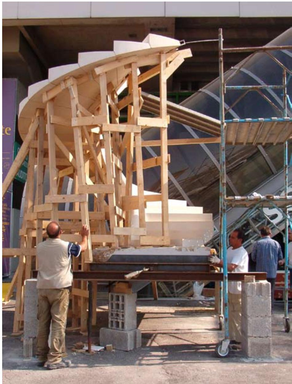
The challenge, from a research point of view, was to design and calculate a stone structure composed of discontinuous elements submitted to precompression through the post-tension of a harmonic steel cable in a helicoidal system. Unlike normal structural praxis, the structure was not assembled flat, but suspended, thus increasing the difficulty of calculation considerably.
