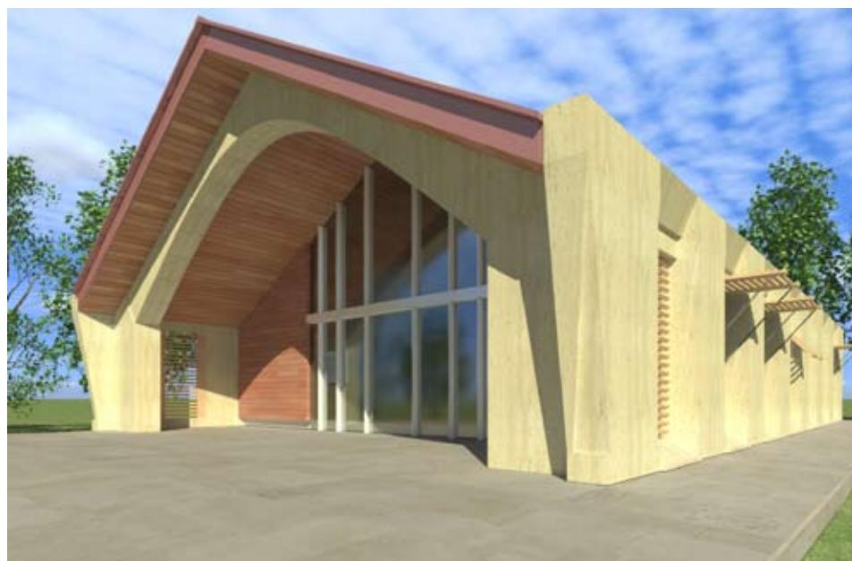
The East and West-facing sides of the house are characterized by the rhythmical spacing of the heavy stone vertical structures that support the arches, creating a monolithic effect.
