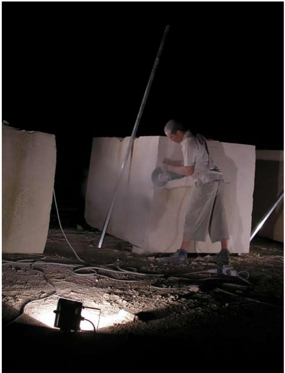
Another element of interest from the point of view of statics, is the suction effect created between the joints . The perfect joining of the blocks caused a pneumatic suction effect that, functioning as a 'glue', theoretically obviates the need for cables to reinforce the structure. This prototype represents a constructive solution of great interest in the construction of large pillars or stone columns.
